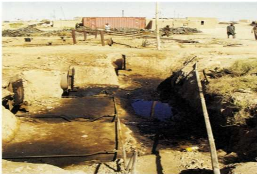
Boilers leaking crude oil onto the ground at Shiburghan
