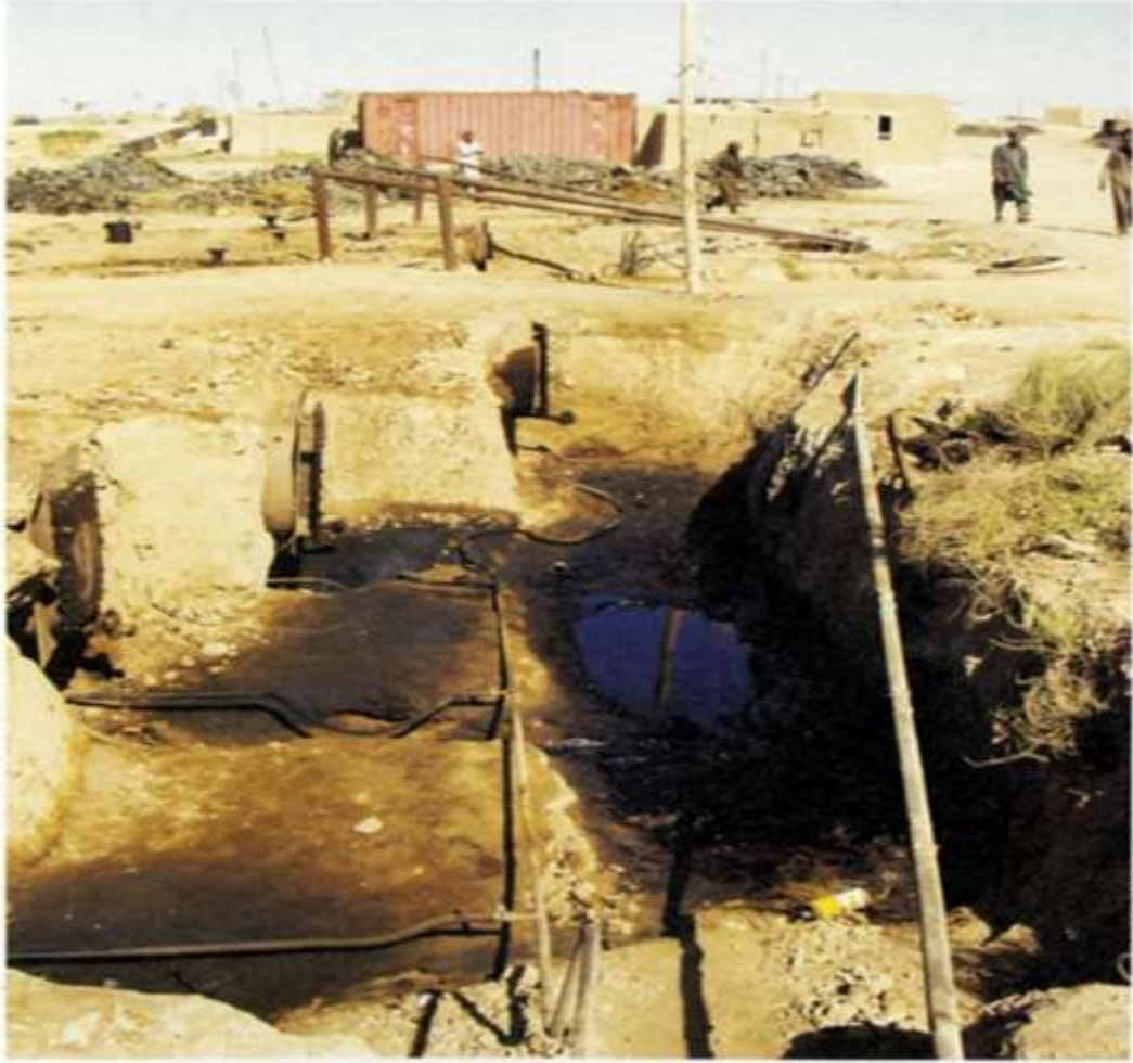
Boilers leaking crude oil onto the ground at Shiburghan
