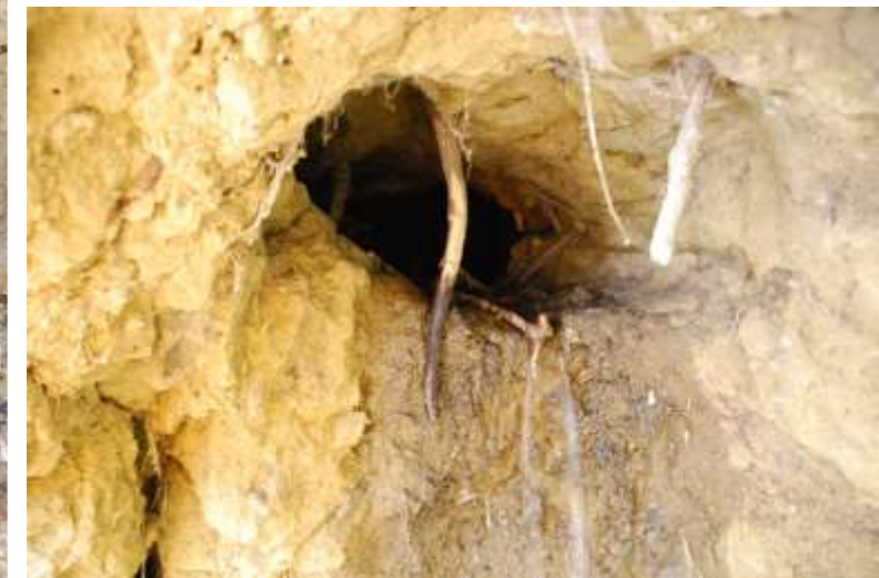
Piping exits Loess Hills, Iowa
