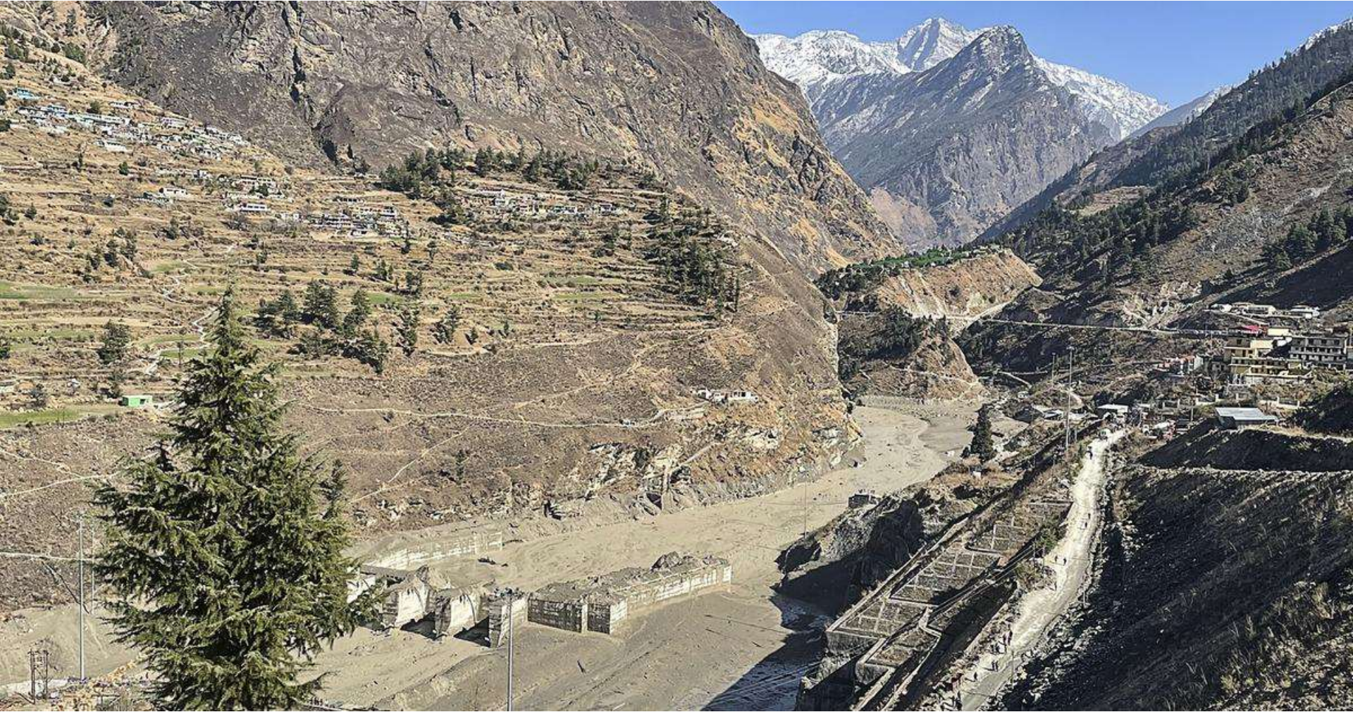
Rishiganga Hydroelectric Project and dam
