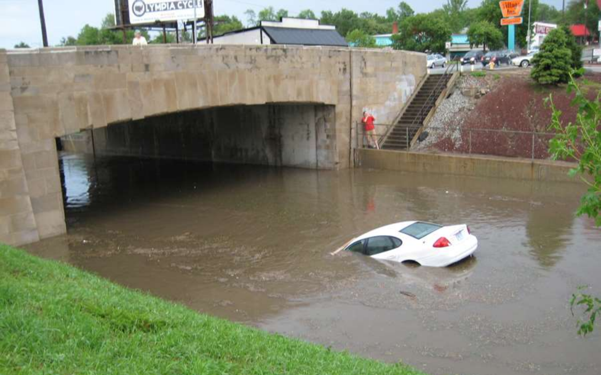
Saddle Creek “Road” and Dodge Street Bridge – June 27, 2008
