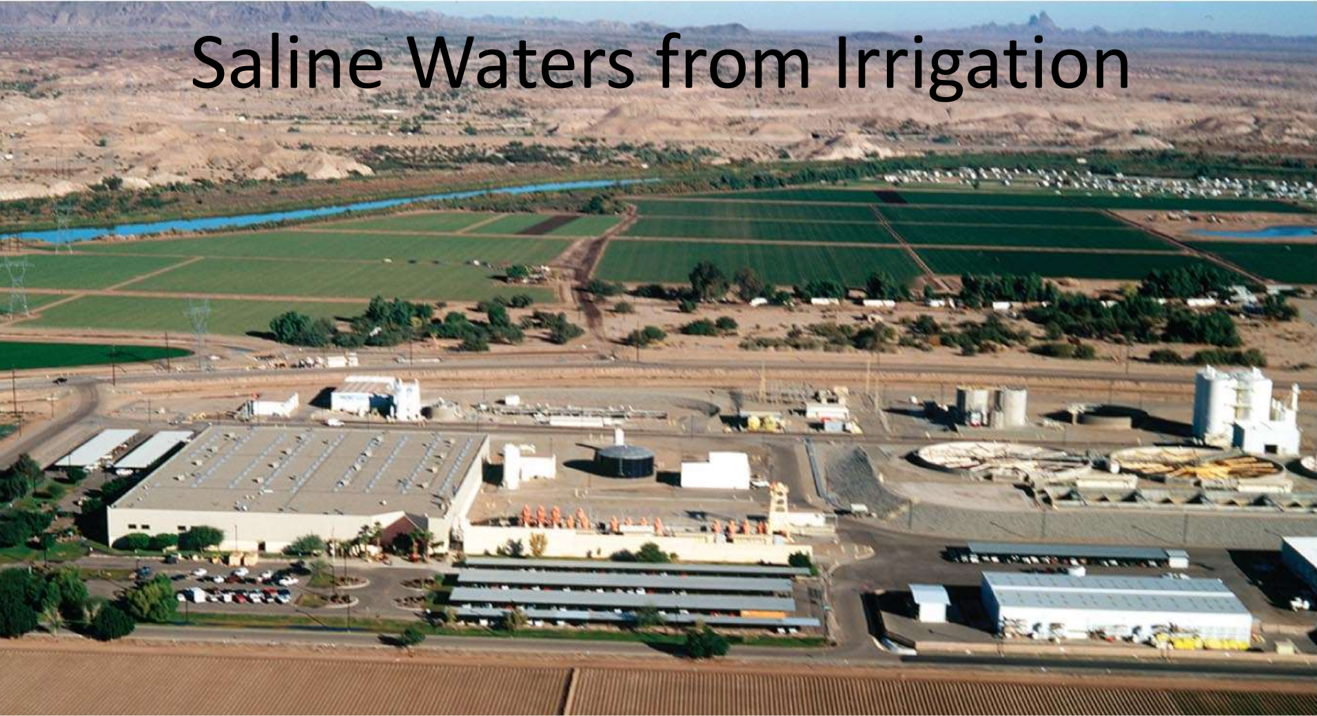
Figure 10-6 The Colorado River Desalination Plant
